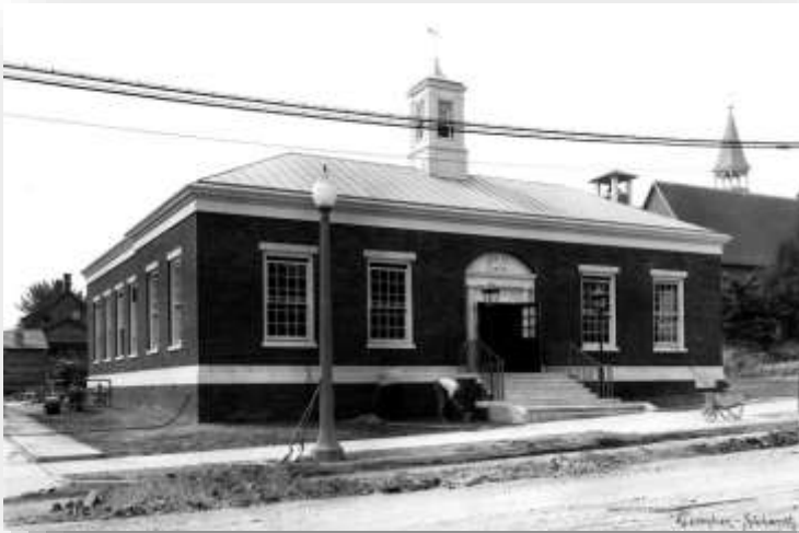
Old Snohomish PO (now city hall), built 1937, faux colonial
